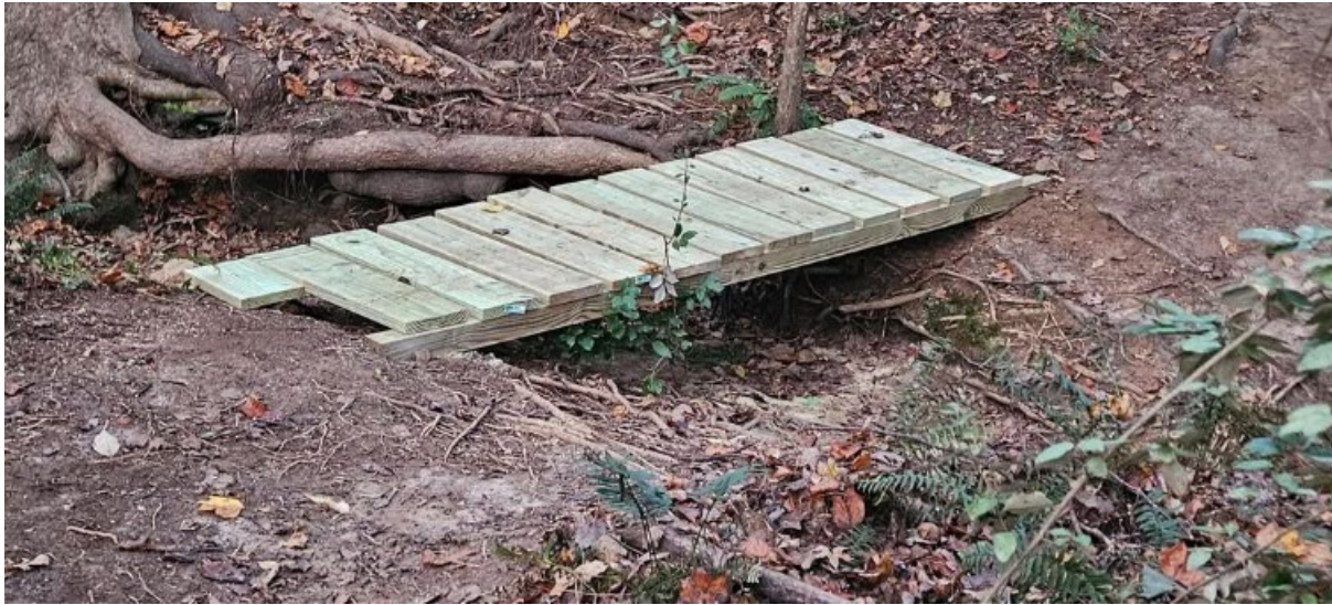
Figure 14. Example Photo of an example of Basic Plank Crossing – low impact construction
