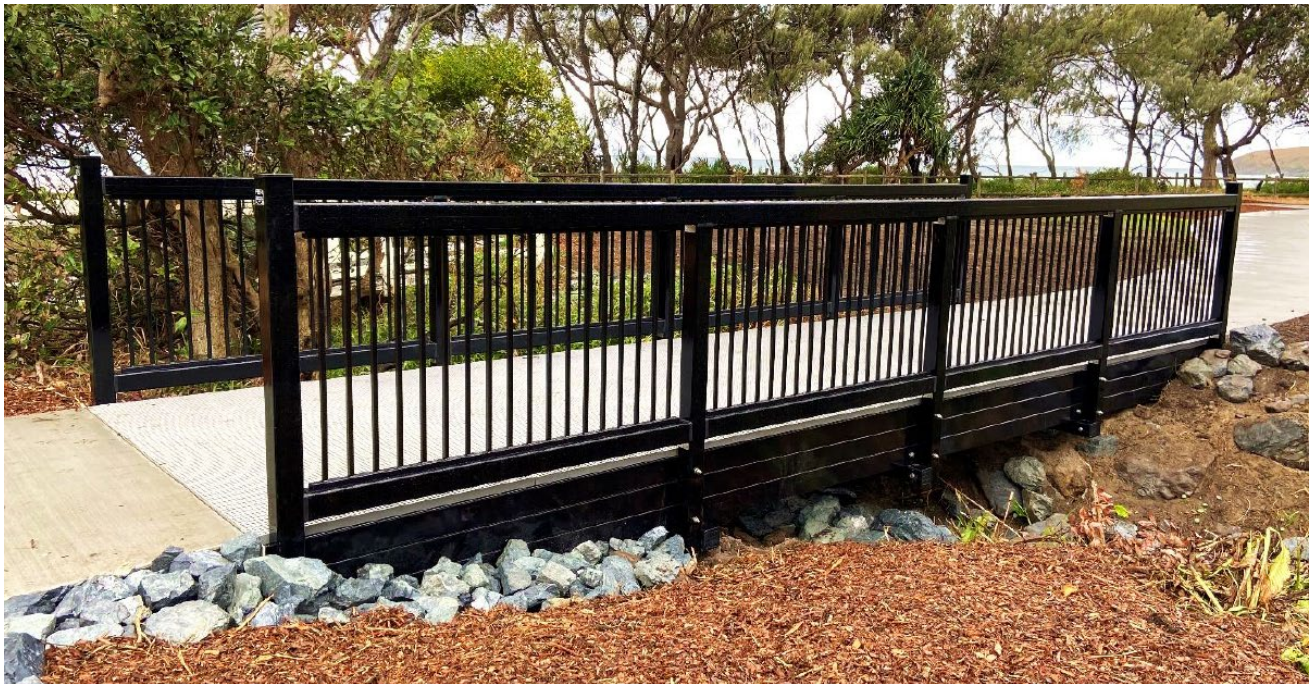
Figure 15. Example proprietary FRP Height Safety Bridge
